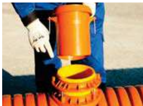
8 Inserimento codolo 8 Application of socket
