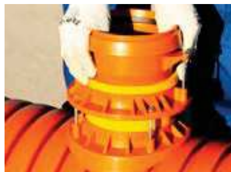
9 Serraggio viti autofilettanti 9 Tightning of self-tapping screws
